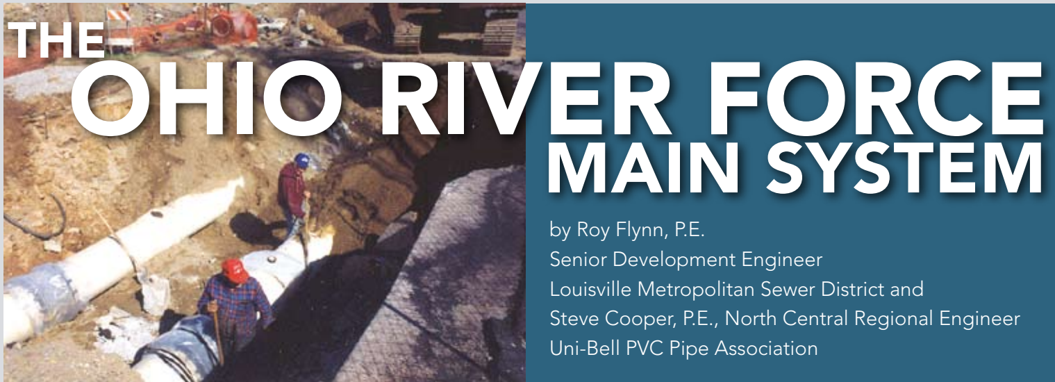
Dual, 24-inch, PVC sewer force main.
