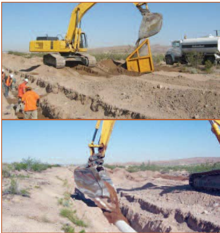
Figure 6. The embedment was screened (top) to remove cobbles and boulders from the embedment material. The embedment was placed in loose lifts of 24-inches (bottom).
