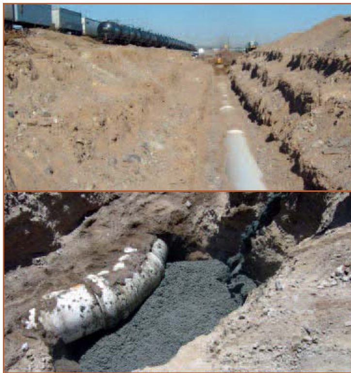
Figure 7. Portions of Reach 4A paralleled active railroad tracks (top). The huge forces generated at changes of direction in a 24-inch pipeline required enormous thrust blocks (bottom).
