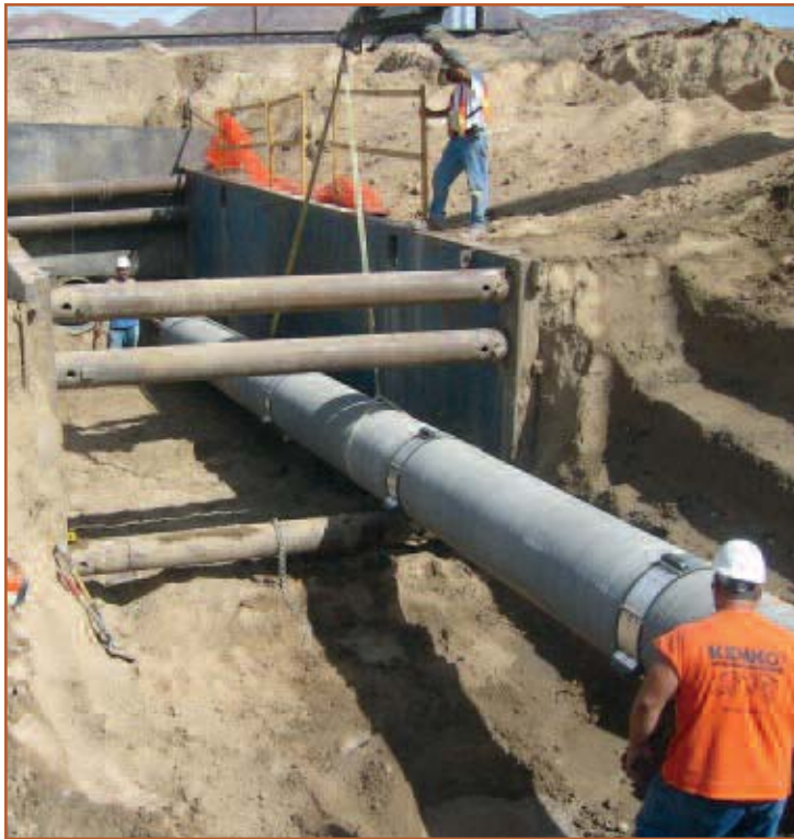
Figure 4. Cement lined and coated steel pipe had been the MWA's pipe material preference. This type of pipe was used for the first three reaches of the MRPP. This photo demonstrates the skill of the backhoe operator, who is threading the steel pipe through the braces of the trench box. Bumping the pipe against the trench box could be disastrous for the internal and external coating. As indicated by the casing skids, the pipe is to be pushed into place inside a casing.
