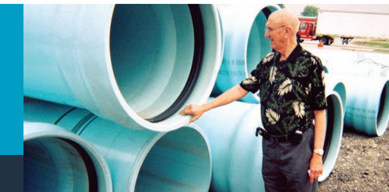
Fred Valenta, with JC Utilities, admires the 36-inch PVC pipe being used to replace the ductile iron pipe.
