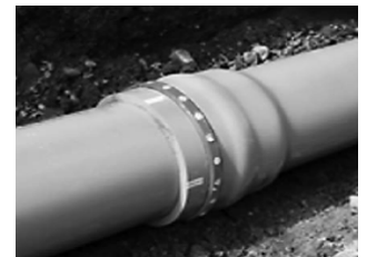
Pin-and-Groove Gasketed Joint
