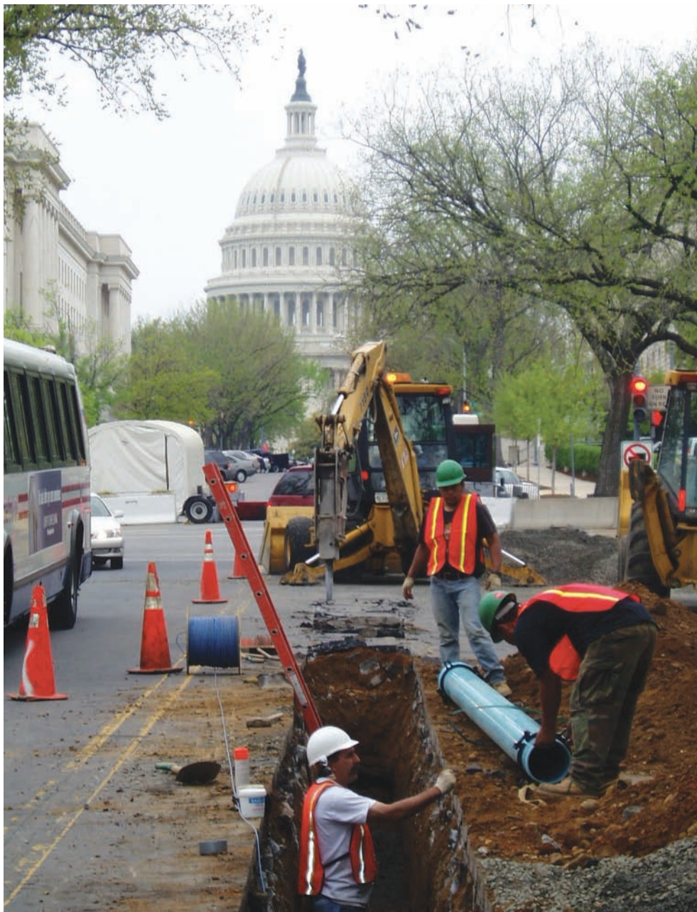
Fort Myer Construction workers install 8-inch PVC water main in downtown Washington D.C.
