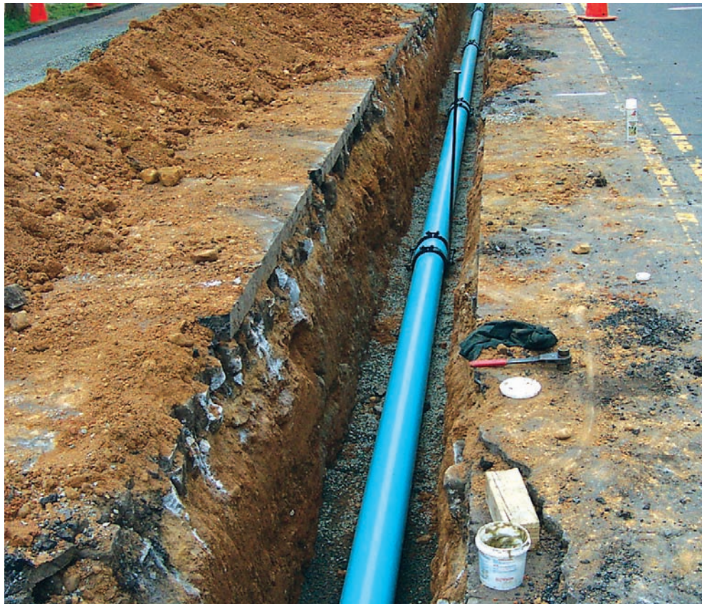
Figure 1b. The 8-inch PVC replacement mains were installed "quickly and smoothly" four-feet below grade.
