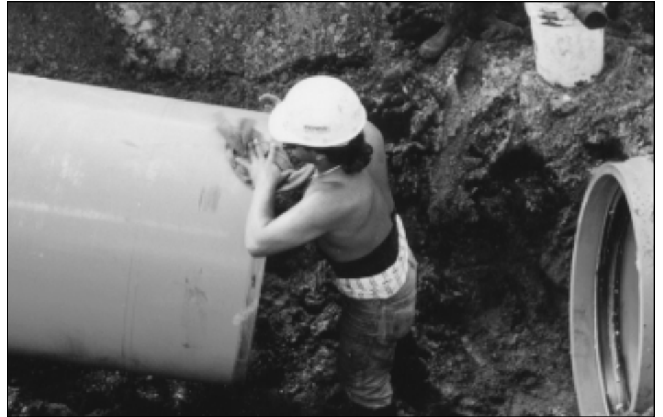
Worker preparing 36" DR25 for joint assembly.
