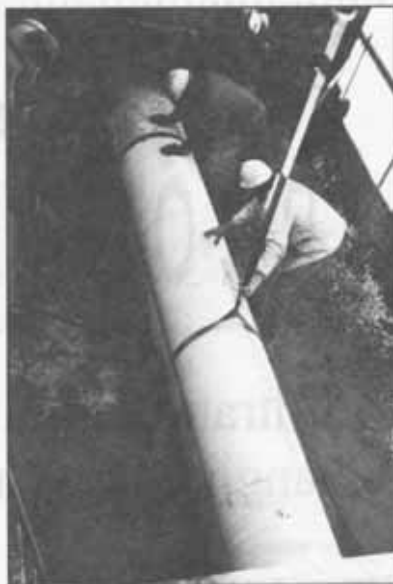
Joint is lined up for quick coupling and insertion.
