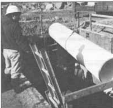
Slipline lowered into shored insertion pit.
