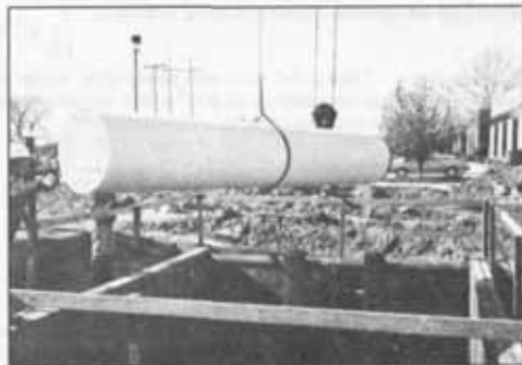
High impact toughness and longitudinal stiffness contribute to PVC slipliner pipe's ease of installation.
