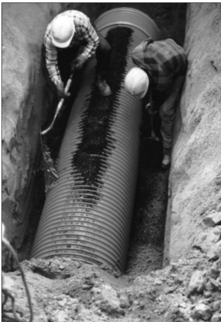
Workers shown shaping and placing material for bedding pipe.
