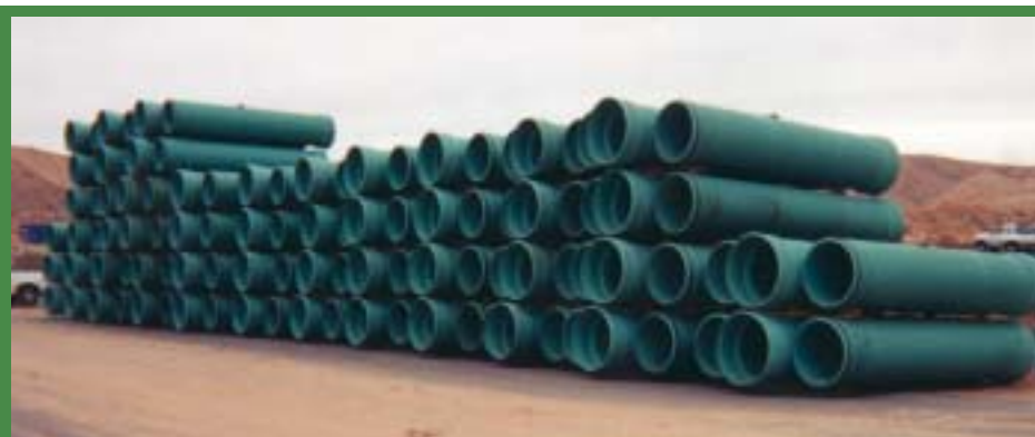
Delivery of the 30-inch profile pipe was critical. The downtime of the irrigation supply had to be minimized for these desert golf courses.
