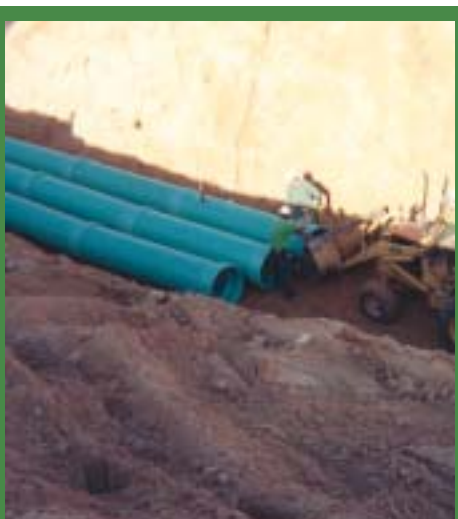
The trapezoidal ditch ranged in depth from fifteen- to twenty- feet deep. The top width was up to fifty feet wide.
