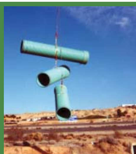
Slings of differing lengths reduced handling time of the triple-barrel installation.
