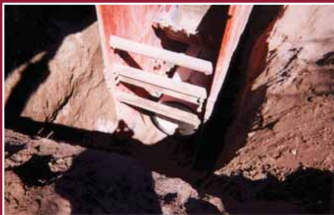
The nylon sling was rigged as a choker around the sewer pipe and connected the backhoe. Tight space necessitated this approach for joint assembly.
