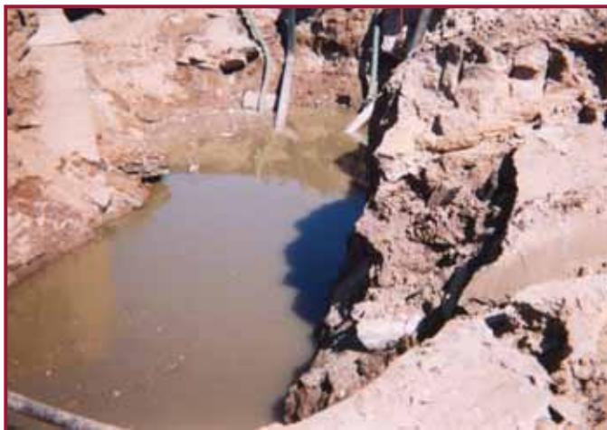
The sink holes were fifteen to twenty feet deep. Pumps were brought in from across the southwest to clean-up the spilled sewage.
