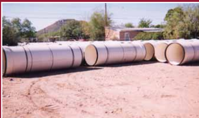
Two loads of 48-inch, F1803, sanitary sewer pipe were delivered three days after it was ordered.
