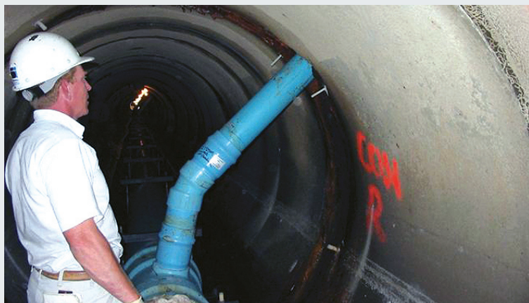
Sanitary sewer Laterals were reconnected as the work progressed.
