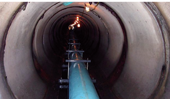
Avon Lake's unique solution for separating a combined sewer.
