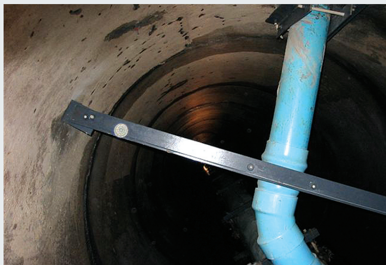
Bolts, rods, and brackets were made of reinforced nylon to keep the entire system non-metallic and corrosion free.
