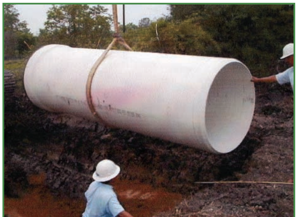
The longer lengths of PVC and its lighter weight reduced the installation time when compared with RCP.
