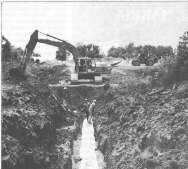
Major new industries required the installation of a new force main.
