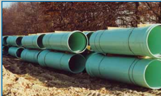
This project required 34,000 feet of 36-inch F679 pipe.
