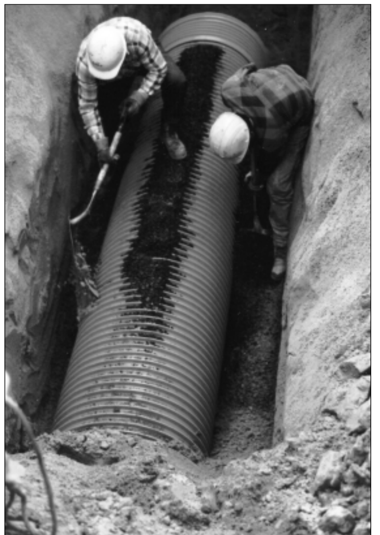
Workers shown shaping and placing material for bedding pipe.
