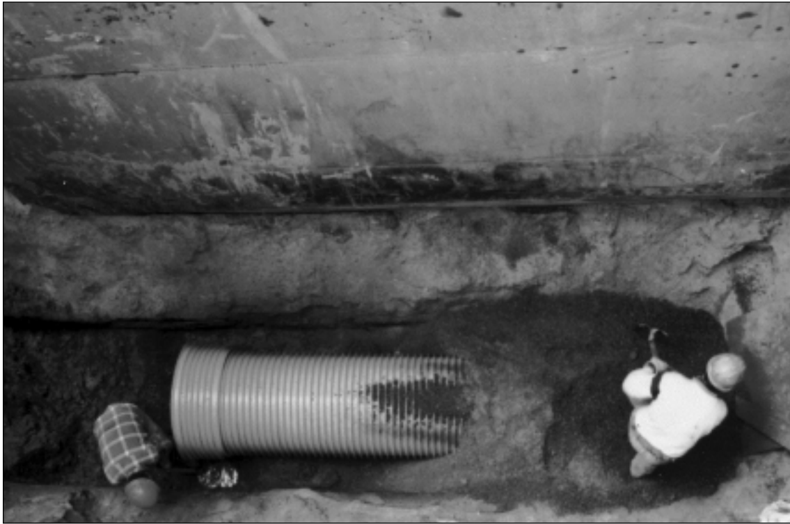
Trench boxes were stacked for this deep installation. Import material is shovel sliced into the haunches.
